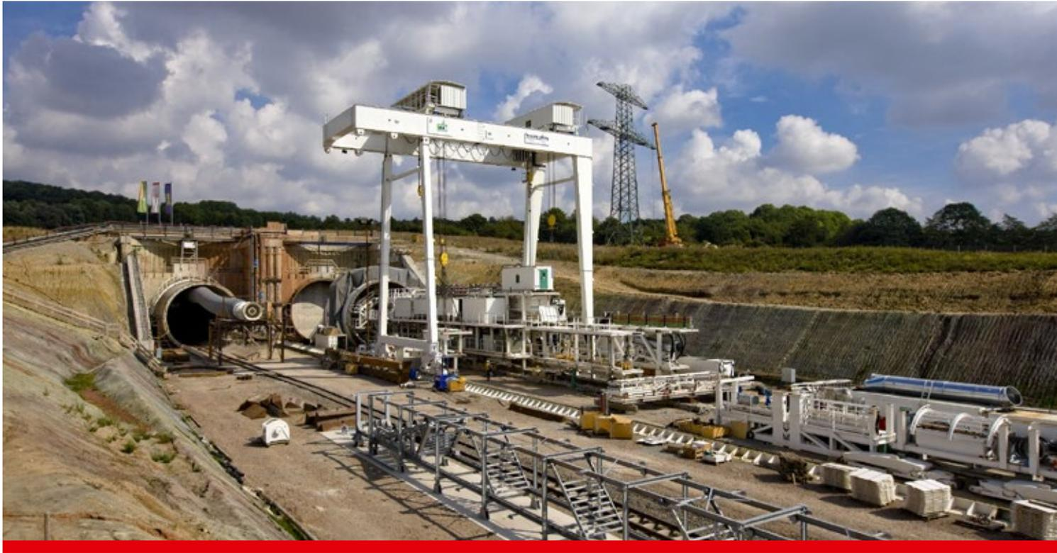
The 8,280 meter long Finnetunnel in Thuringia was realized by the Tunnel Construction Division as Co-TGF (technical leadership) with two convertible Mixshields Hydroshield in closed and open mode for DB Netz AG.
