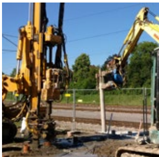
Vertical drilling of freeze pipes
