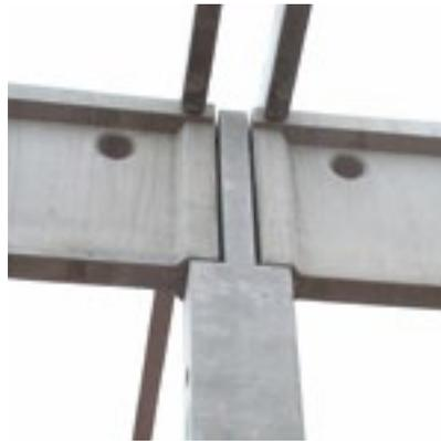
*Special prefabricated elements made of steel fibre concrete were used for the construction of the two to four-aisle halls.*
