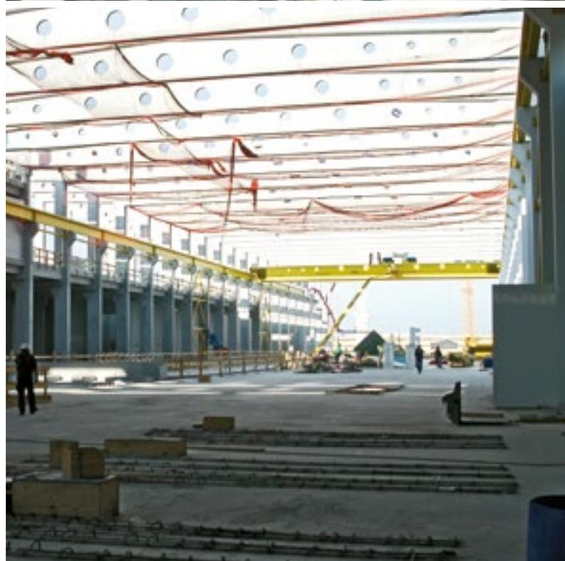
*Within only six months of shell construction time, around 7,000 high-quality, prefabricated concrete units were assembled quickly and precisely.*
