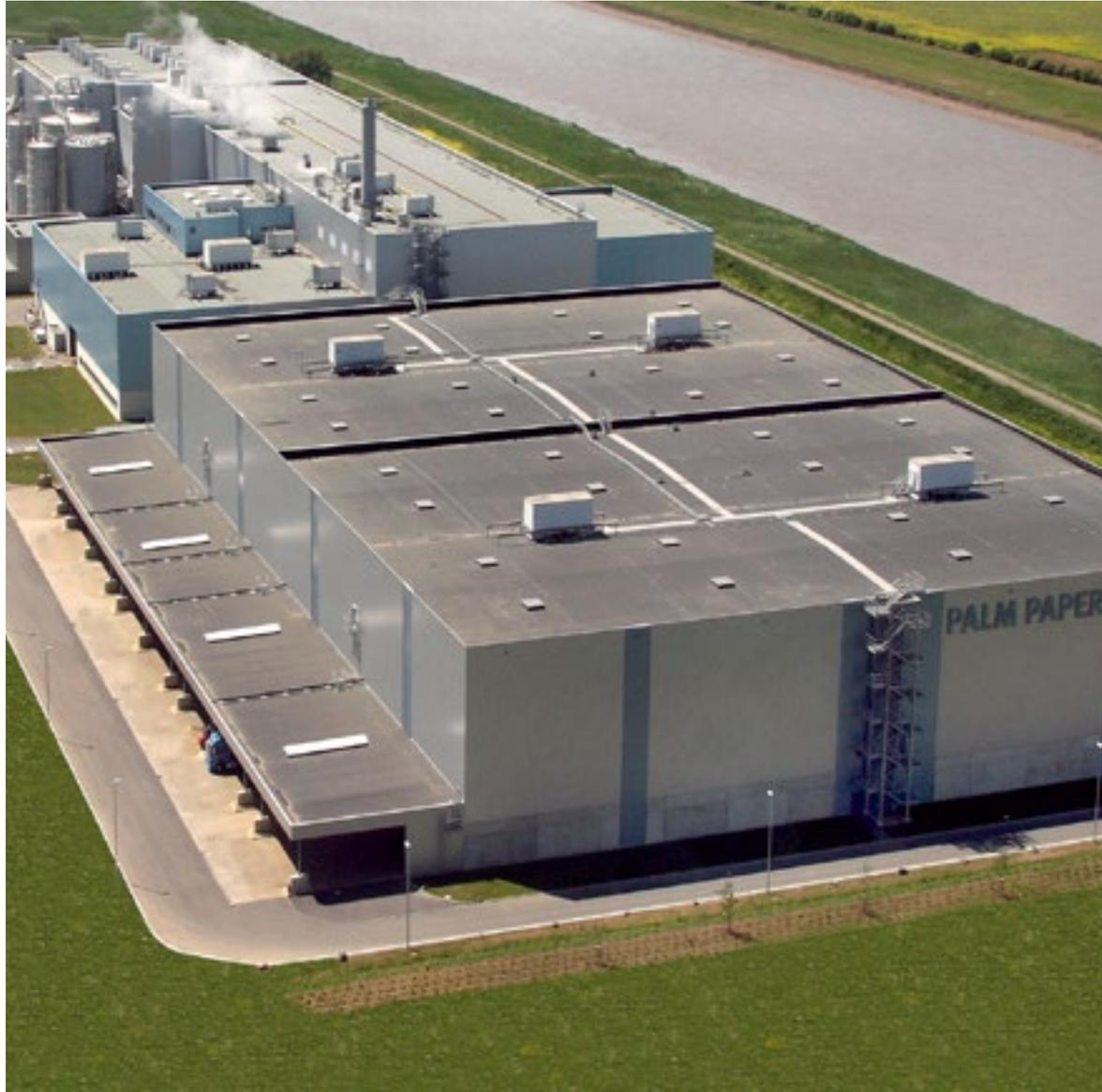
*Over eight months, 10,560 concrete components used in building the paper factory were transported to the site via ship and canal.*
